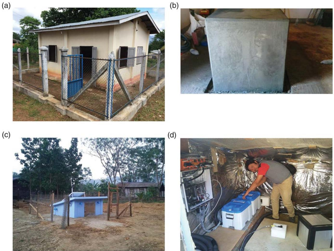
▲ **Figure 3.** Installations of Keng Tung (KTN) and Tamu (TMU). (a) Existing small concrete building in Keng Tung (KTN) with (b) newly constructed instrument pier. (c) Newly constructed vault in Tamu (TMU) and (d) Tamu (TMU) vault interior.
